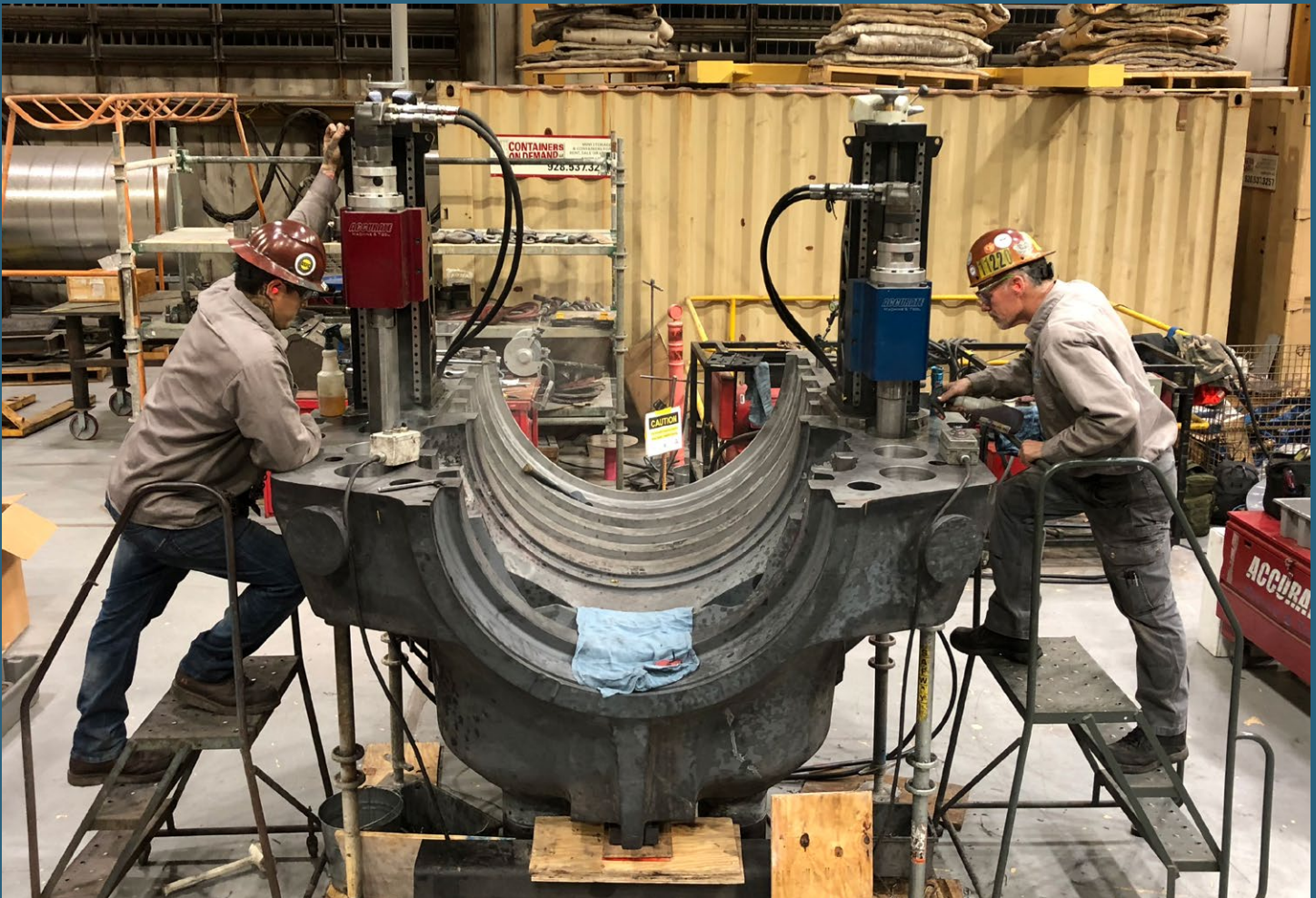
Removal of Studs Oversizing to an 8" Diameter
