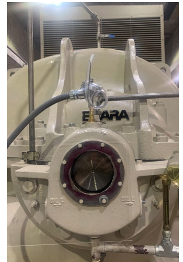
Many of our services can also be performed in the field such as bearing and seal changes
